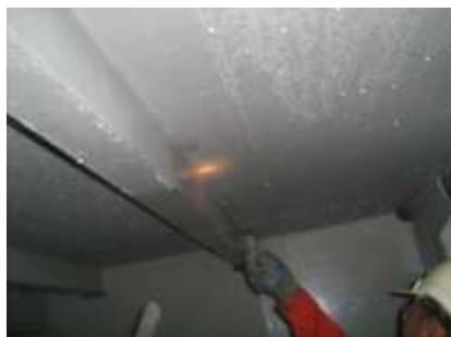
Applying RA 500M in wet surface in a ballast tank
