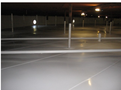
RA 564 applied in crude oil tank BP Dalmeny
