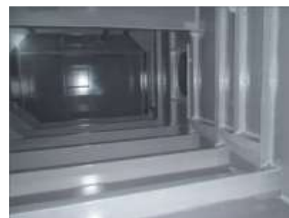
RA 500M applied in a potable water tank
