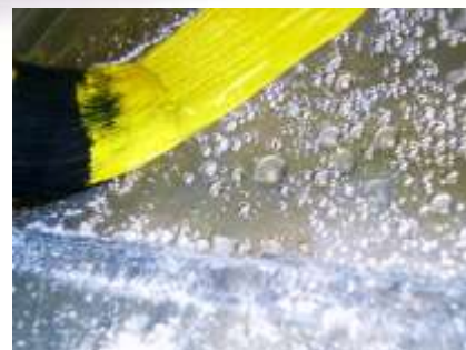
RA 500M - applied to a completely wet substrate
