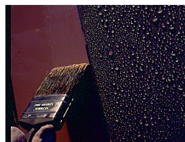
Applying RS 500P on a sweating and wet substrate
