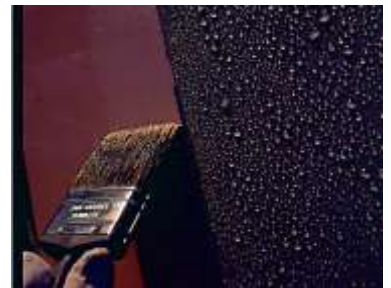
Applying RS 500P on a sweating and wet substrate
