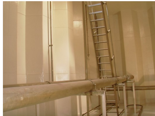
Completed project - 2 x 500µ DFT Chem-tect™ RB 364 applied to a Sa 2½ grit blasted surface
