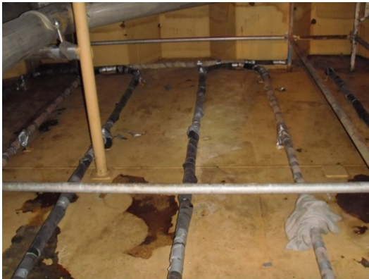
Chemical tanks before cleaning and surface preparation
