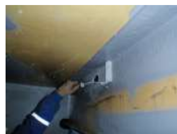
Applying RA 500M on wet surface
