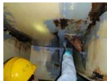
Applying RS 500P on wet & rusty surface
